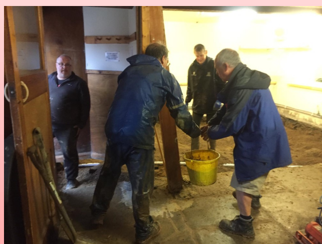
Sally, Andy, Bill and John bucketing in loads of ballast .
