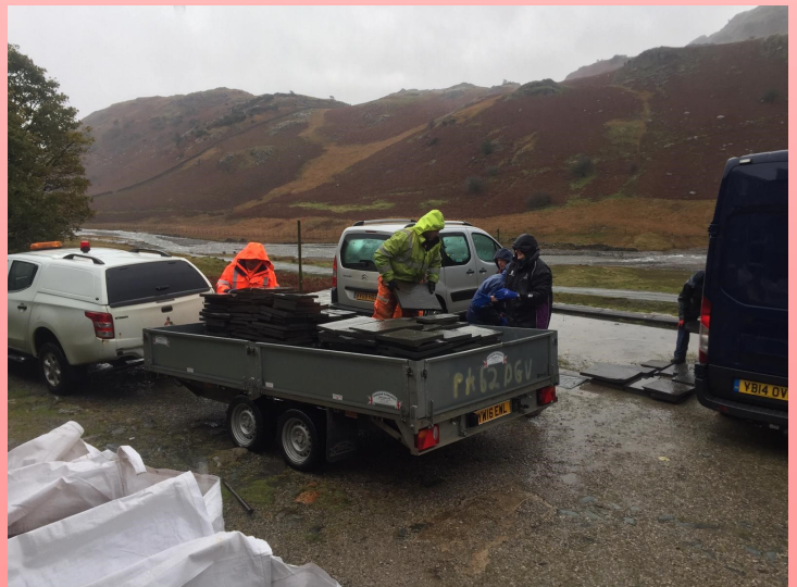
Unloading materials (all done by hand)
