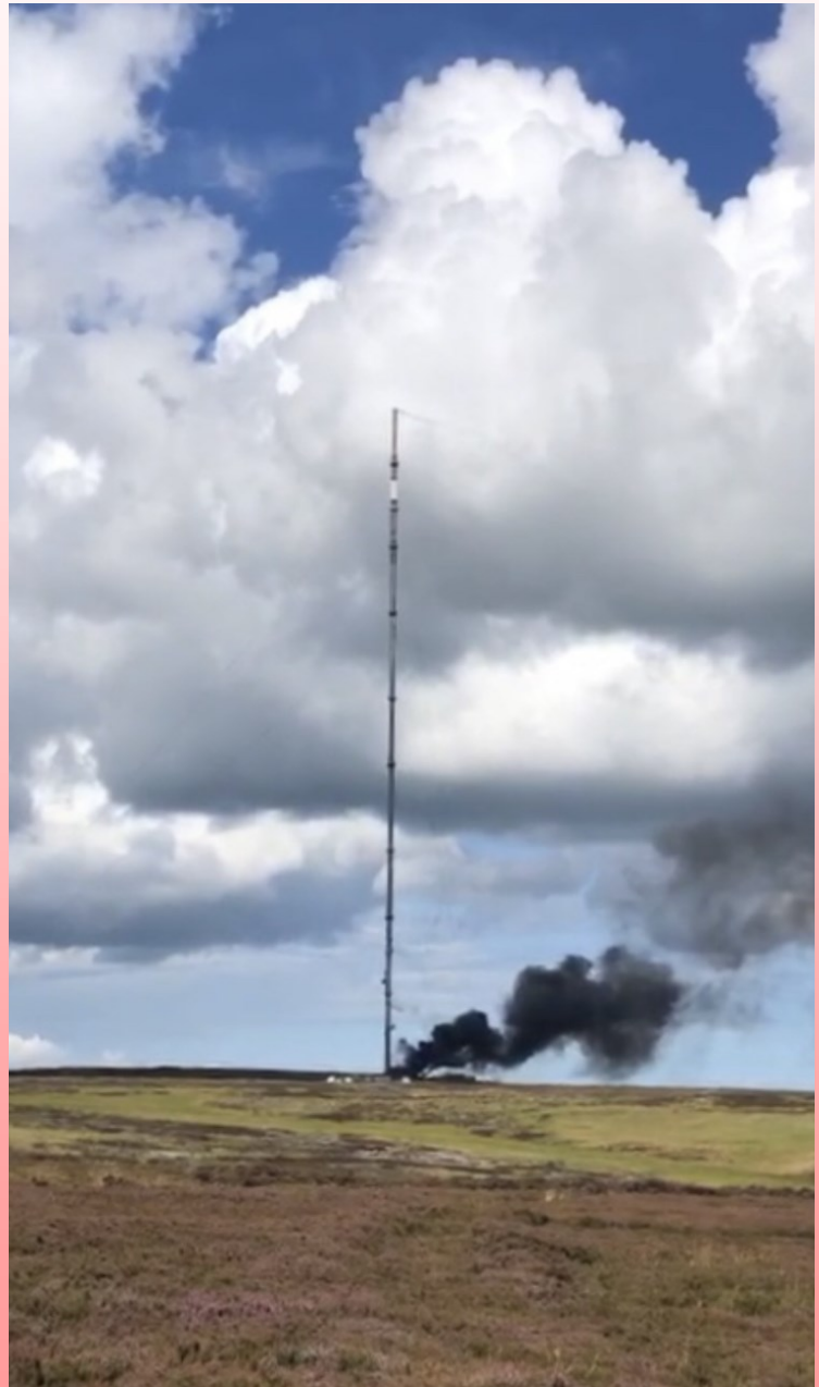
The fire at the original mast on Bilsdale West Moor
